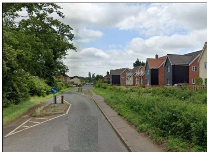
Figure 2.5: Traffic Calming Measure in place
